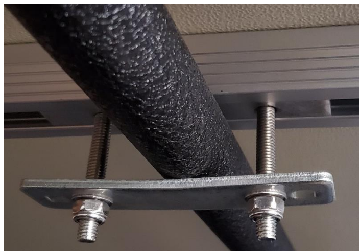
Base plate secured around crossbar on roof rack.
